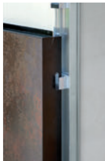
Mechanical anchoring of the connection system (Step 2)
