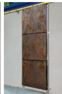
Portion of a finished curtain wall
