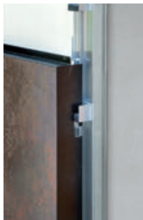
Mechanical anchoring of the connection system (Step 1)
