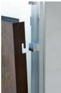
Joining the frame to the substructure
